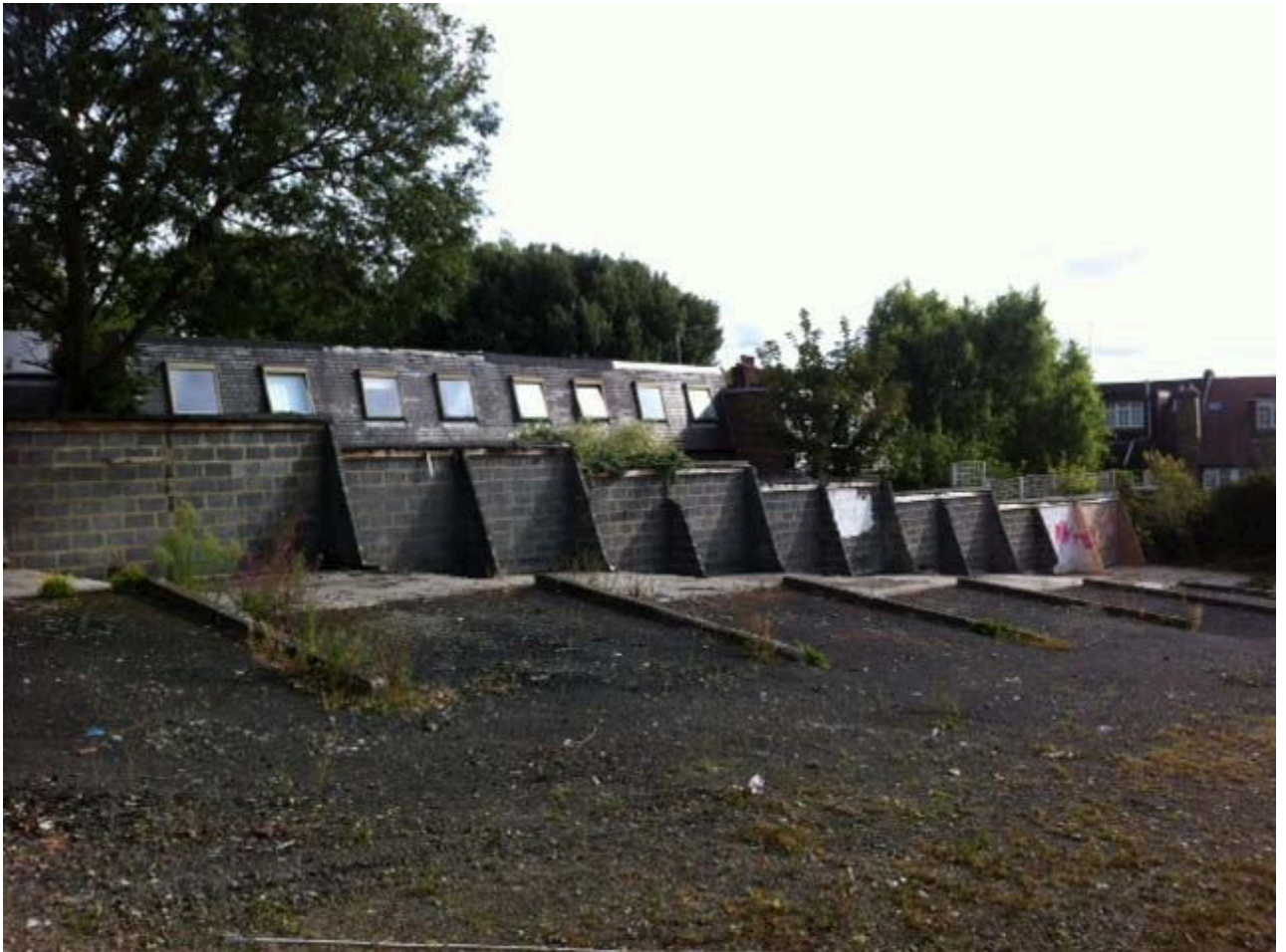
Northern Boundary Wall of Site
